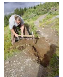
Digging with a # 2 Down
